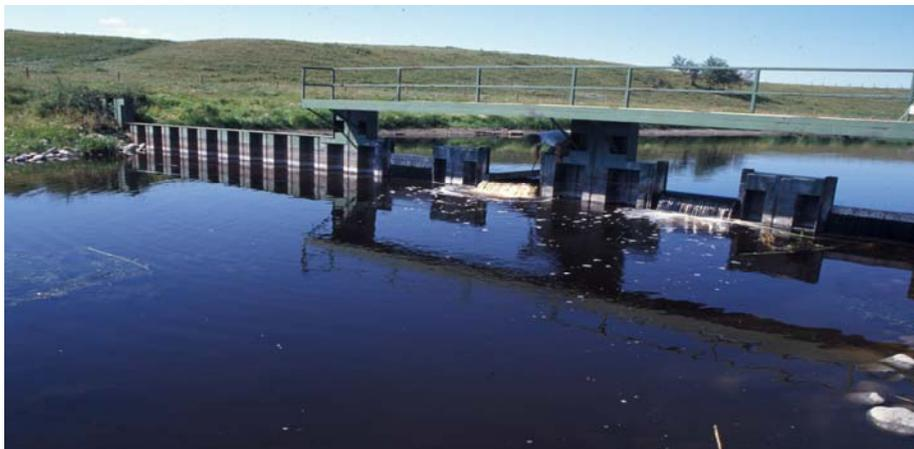
**Variable Crest Steel Sheet Pile Weir**
