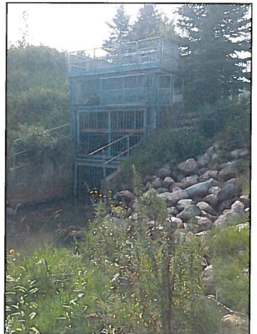
The Mill Creek Ravine oil separator began operations in 2000.
